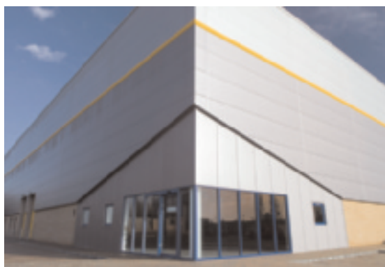
A bespoke warehouse solution on our mixed business park in Ipswich
