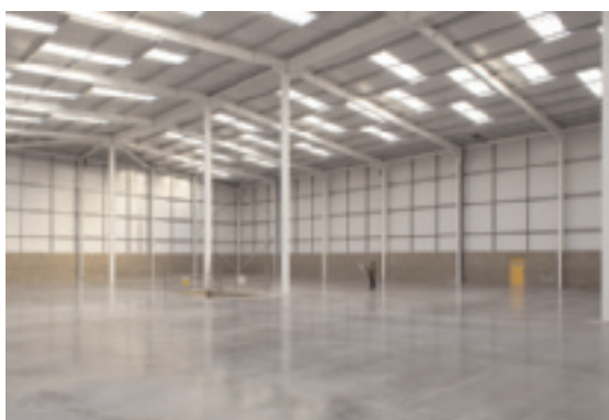
Clear and light industrial space built for our mixed business park in Ipswich
