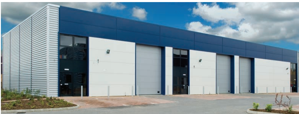
The Black Teknigas building developed by Artisan at Colmworth Business Park, owned by Artisan (UK) Properties Limited.
